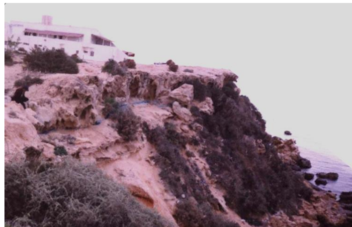
Fig. 1.6: Example of buildings which are sited above the cliff at station no.7 (Sabratah), which will be threatening by coastal erosion
