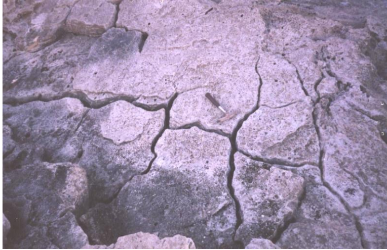
Fig. 3.39: Cracks in Karrot Member (unit 4) at station no. 6 El Matered
