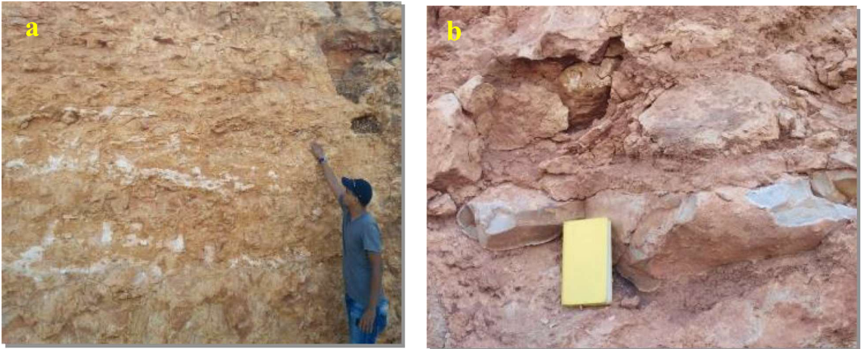
Fig 2.27: a) General view of chert nodules in Darnah Formation; b) close up of the cherts and the host rock as well, (the base of Barsas-Al Hamda roadcut).
