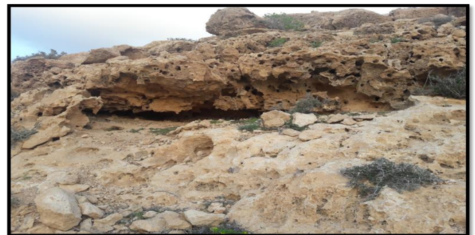
Fig. 9. Honeycomb due to weathering
